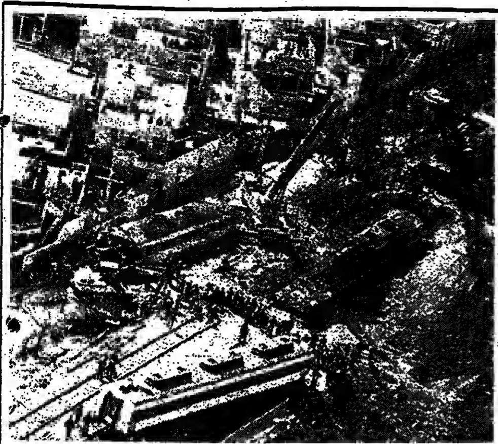
DEADLY DISARRAY —After a cave-in of tracks that killed at least 79 people near the South Korean port of Pusan, passenger cars remained strewn over the tracks. The police said that the cave-in might have been caused by blasting for a tunnel to carry electric cables under the tracks. About 30 meters of track collapsed as the train was moving at normal speed toward its terminal.
